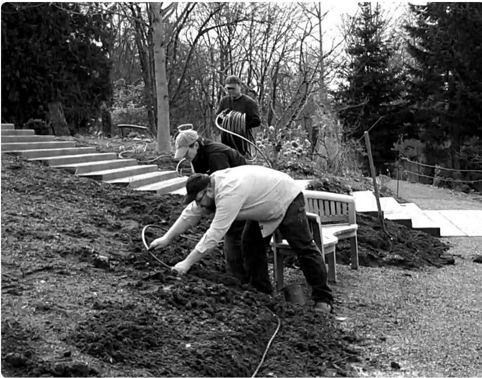
Installing irrigation in the Border in 2008
